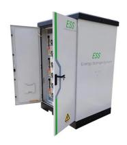
Supply is highly integrated outdoor 5G micro base station power supply system, it combines AC input power ...
