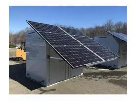
stabilize the photovoltaic output, and a photovoltaic storage system microgrid of a 5G base station is
